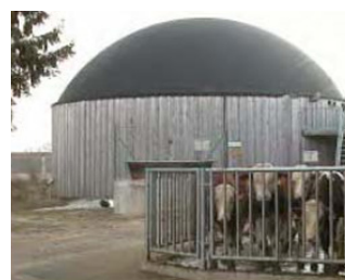
Figure 3: Complete Stirred Tank Biodigester (CSTBR) [12]
