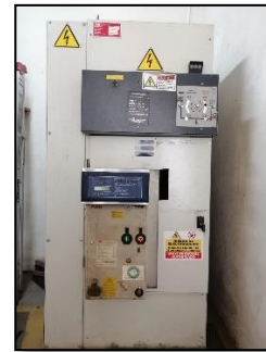
Figura 3: Disyuntor Miami Breaker 17,5 kV/ 630 A/ 95 kV-Bil / Isc 16 kA
